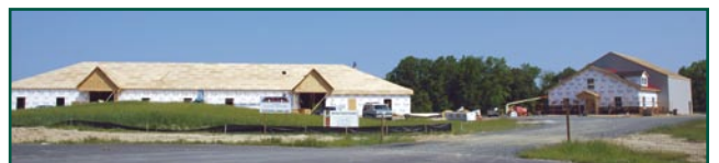
Pictured is a Willow Construction Project at the Talbot Commerce Park.
